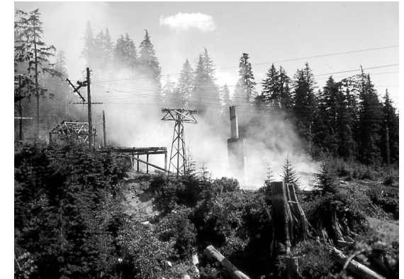
Hi-View Lodge and the top station of the chairlift on the morning after the fire; June 1965 (Alex Swanson Photo)
